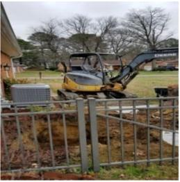
Tests came back and showed the soil around our tank was highly contaminated, so we were moved up high on the priority list. Bay Environmental came out and dug up and removed the oil tank completely. Our engineer said they like to remove them instead of filling them and do so at no extra charge if they are in an area
